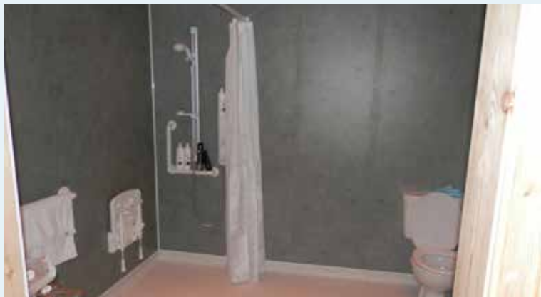
A shower adaptation for a disabled tenant
