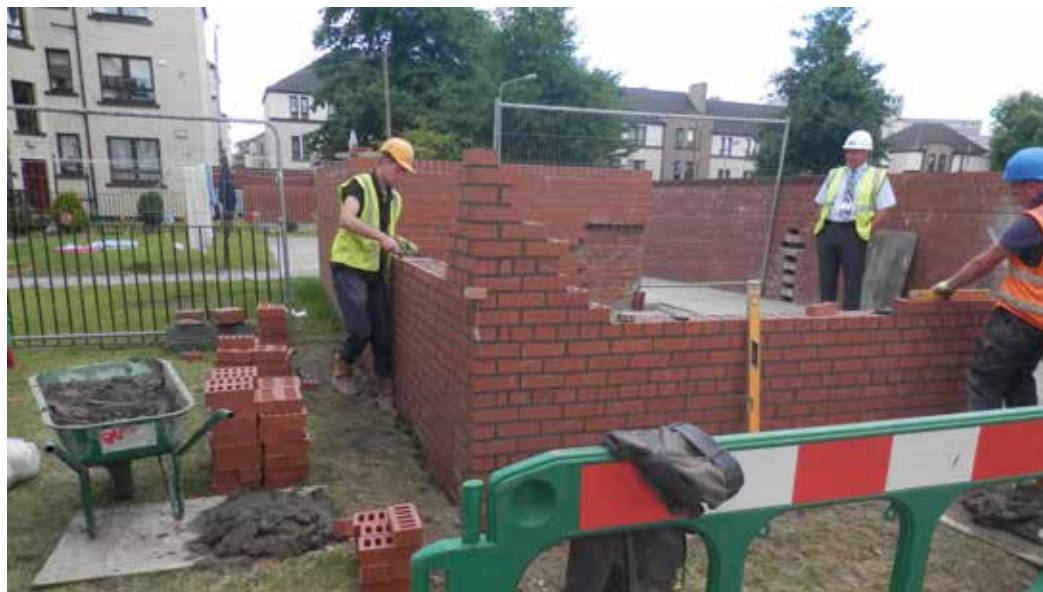
Building a better community...construction work under way
